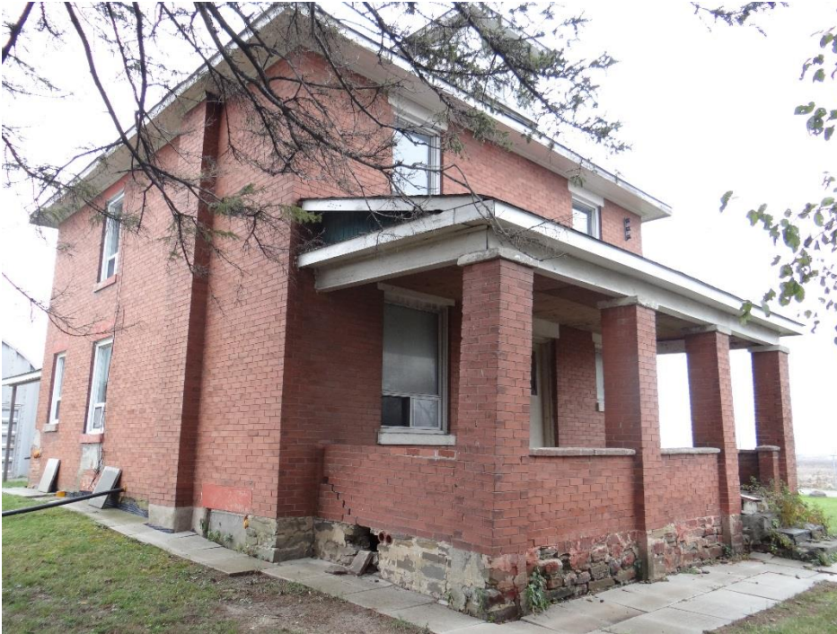
Plate 5: Detail of the stone foundation (northeast corner)
