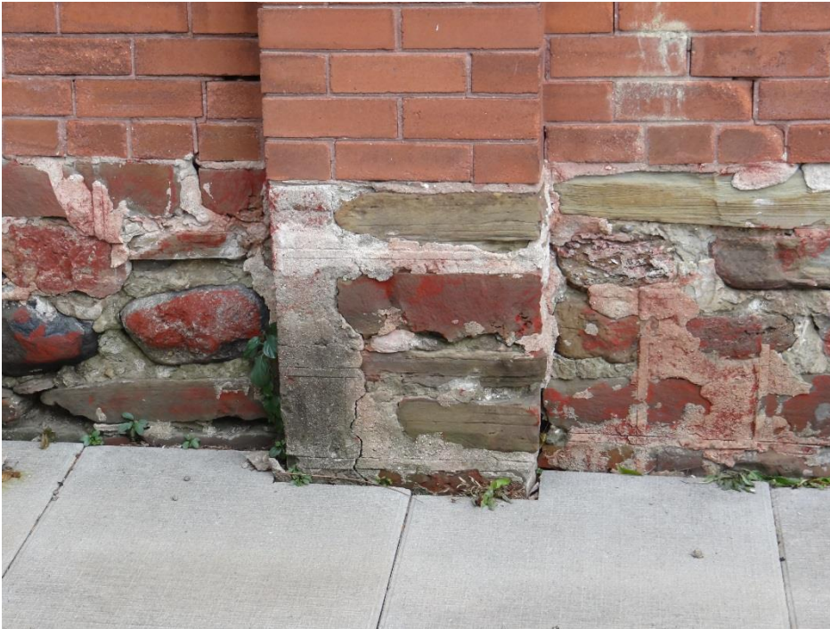
Plate 7: Detail of the stone foundation
