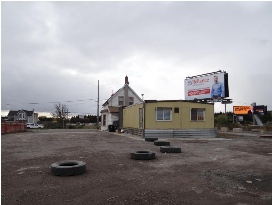
Plate 10: Contextual photo of the north elevation, showing the setting of the building within the property and in relation to surrounding buildings
