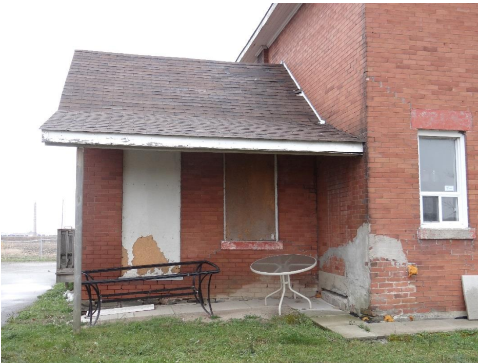
Plate 14: Detail of the rear elevation and parging on the brick
