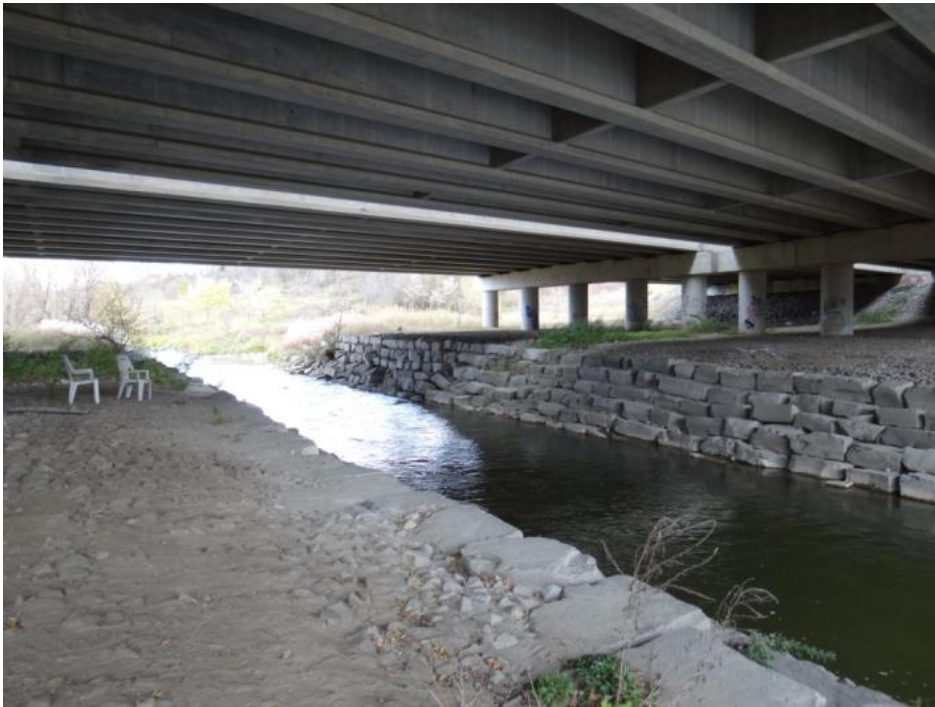
Plate 7: Watercourse beneath the 407 ETR Bridge, looking northeast.
