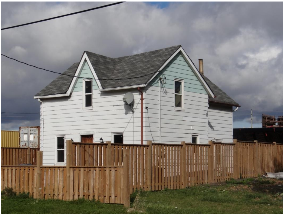
Plate 2: South and east elevations
