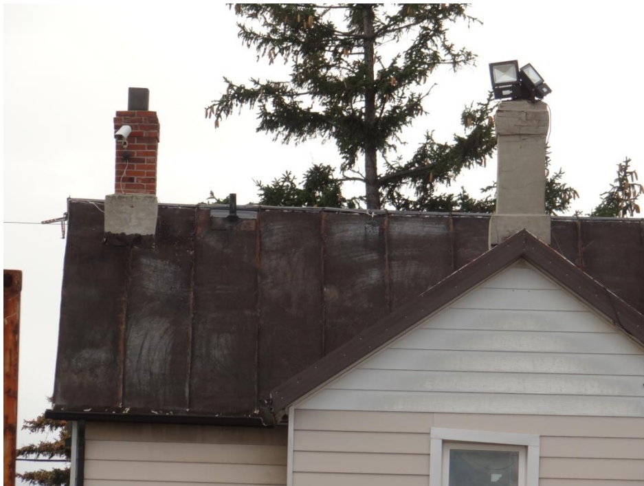
Plate 6: Detail of the roof and chimneys
