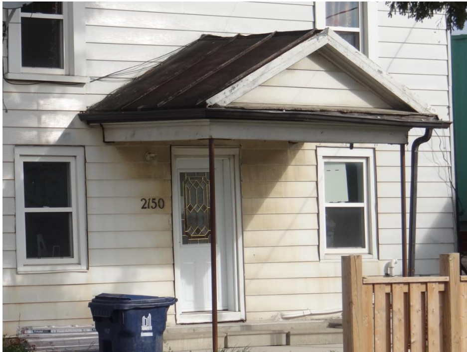
Plate 5: Detail of the front porch
