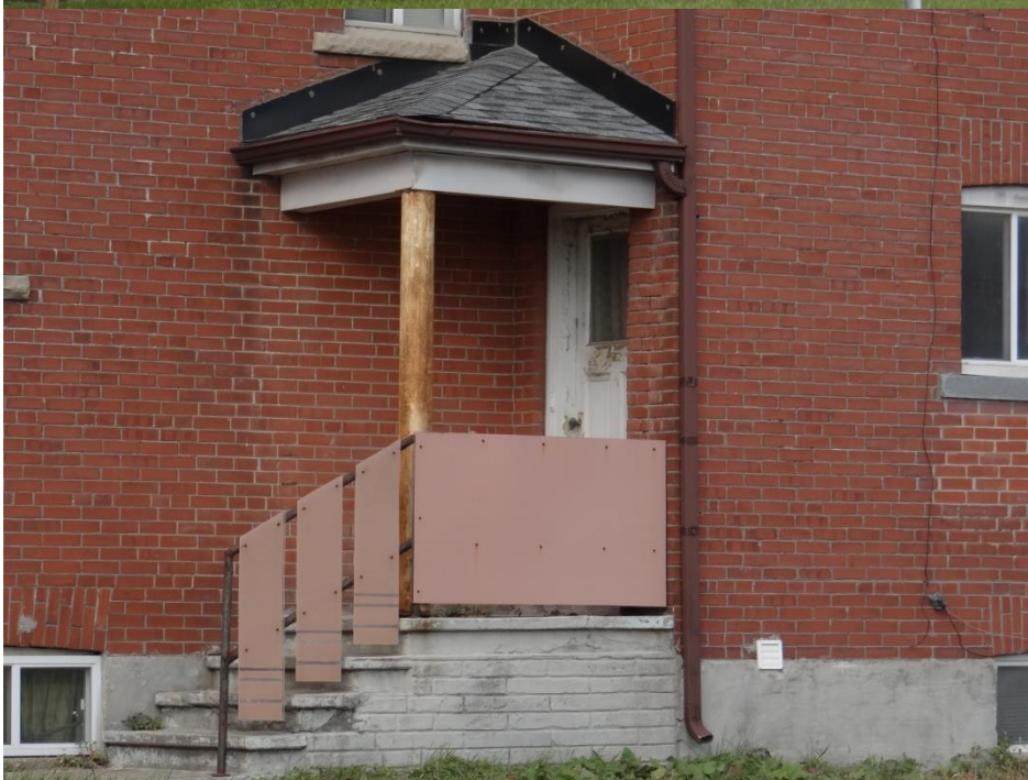
Plate 6: Detail of the side entrance
