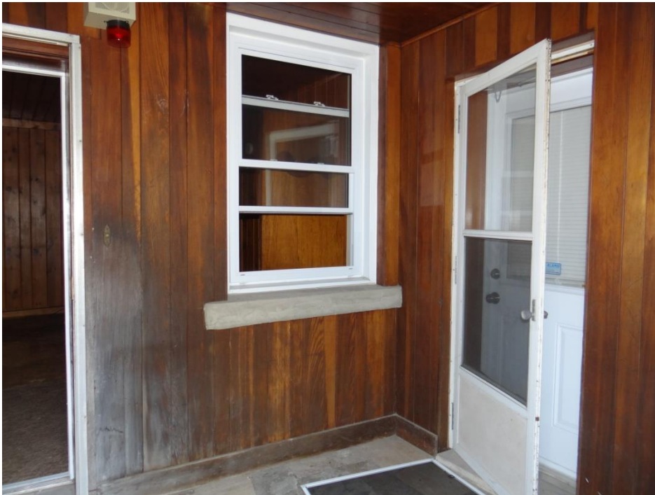
Plate 17: Northeast corner of the mudroom
