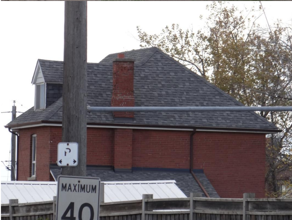
Plate 8: Detail of the roof and chimney
