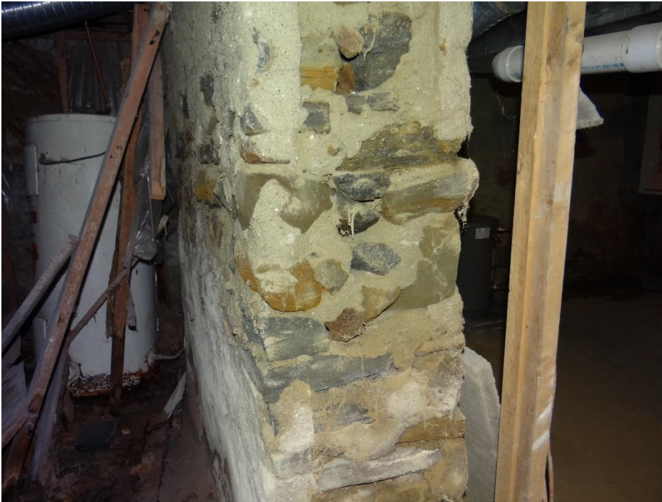
Plate 27: Detail of the foundation
