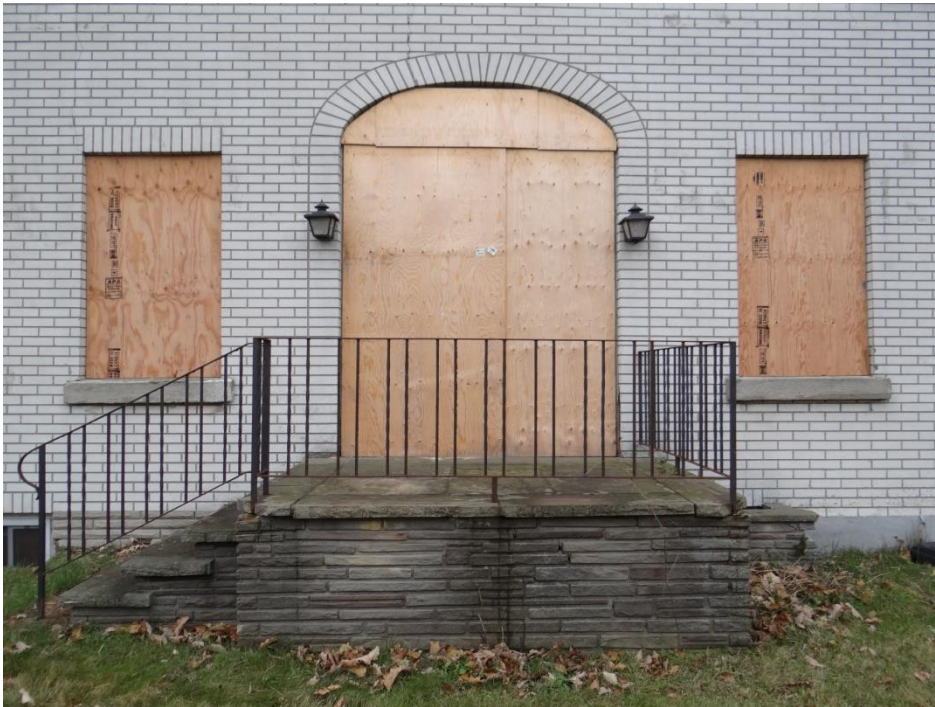
Plate 5: Detail of the first storey of the front (east) elevation. Windows are typical to the house
