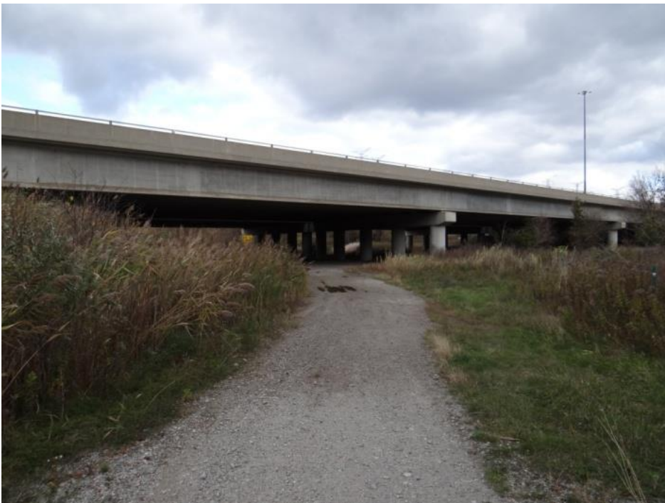
Plate 6: 407 ETR Bridge over the Humber River, looking north from the west bank.
