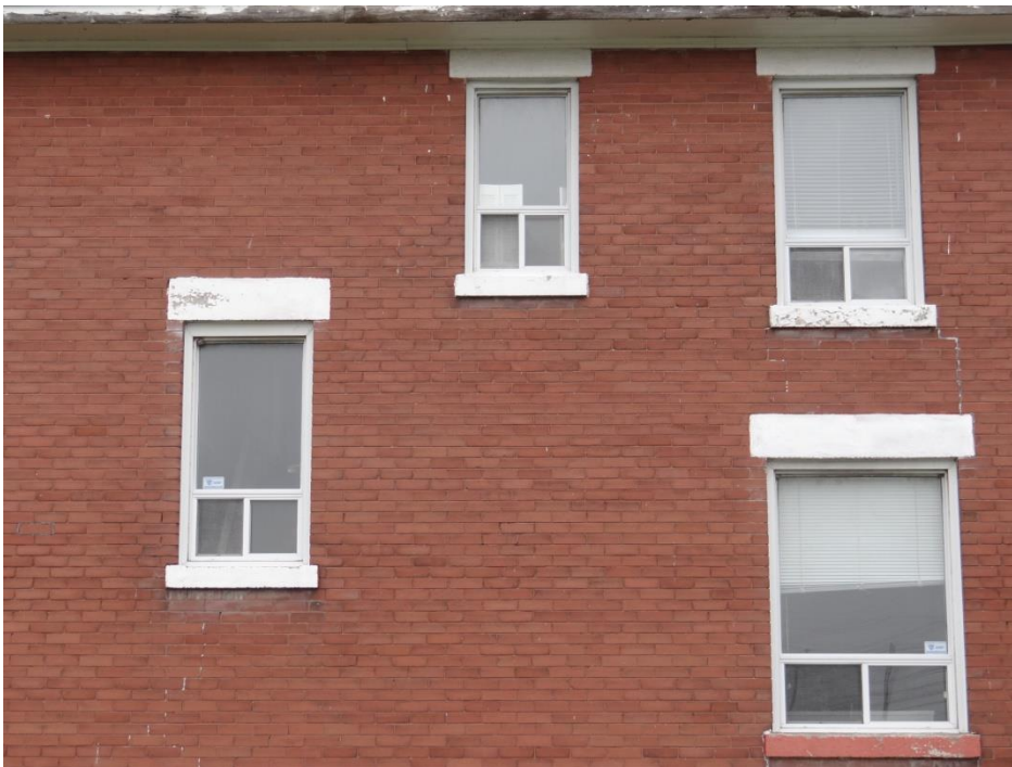
Plate 10: Detail of the fenestration on the south elevation
