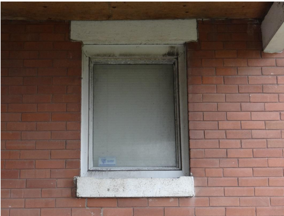
Plate 8: Detail of the window on the front elevation
