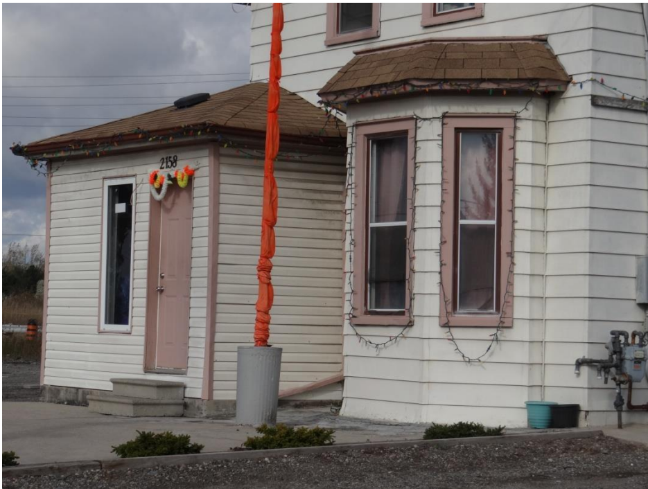
Plate 6: South elevation bay window and entrance
