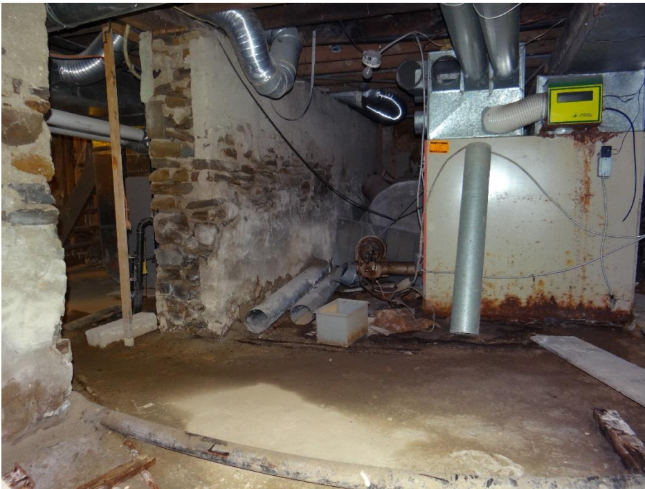
Plate 26: Basement showing fieldstone foundations
