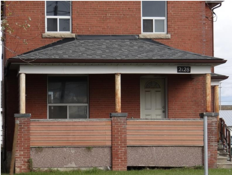
Plate 5: Detail of the porch
