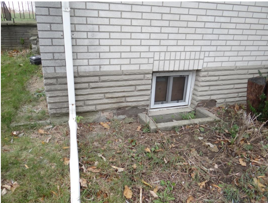
Plate 6: Detail of the foundation, brick and typical basement window (northeast corner)
