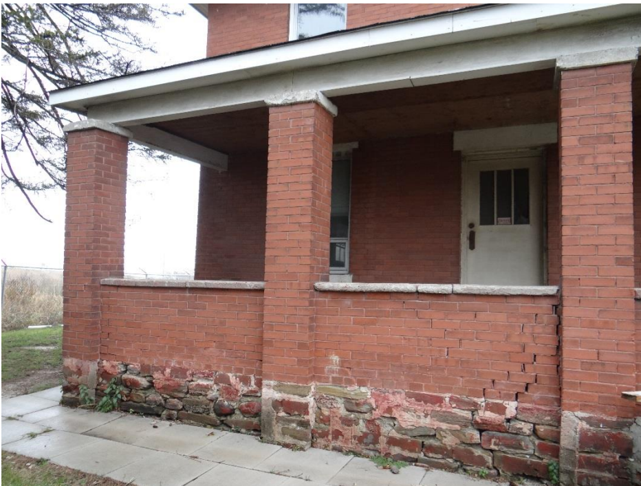
Plate 6: Detail of the veranda and stone foundation
