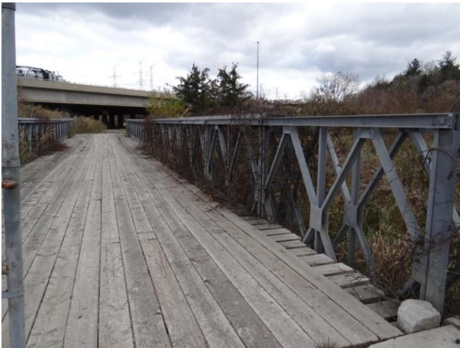
Plate 10: Small bridge carrying trail over western tributary, looking northeast.
