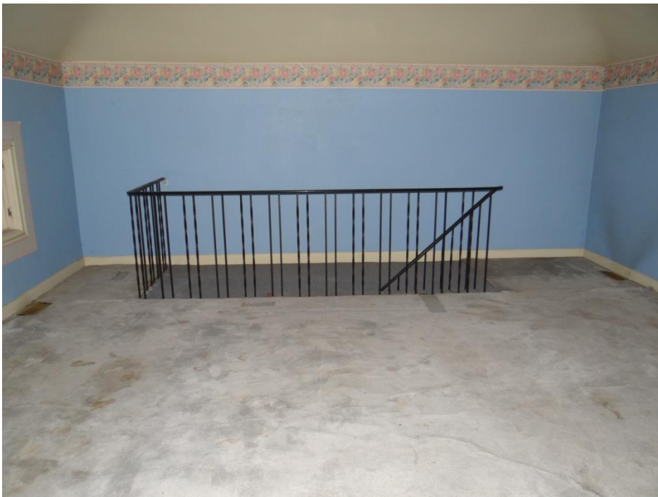
Plate 20: Second storey bedroom in the tail portion showing secondary staircase
