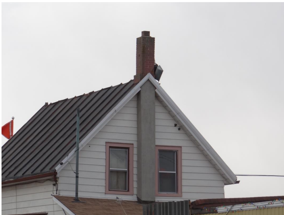
Plate 8: Detail of roof and chimney
