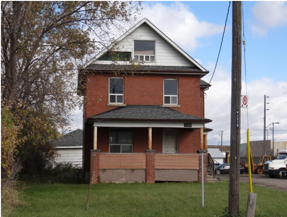
Plate 1: Front facade (south elevation)
