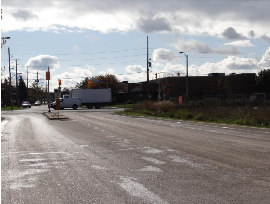
Plate 1: Intersection of Codlin Crescent and Albion Road
