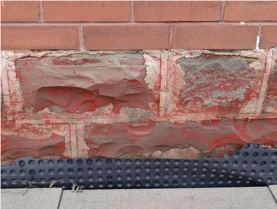
Plate 11: Detail of the foundation
