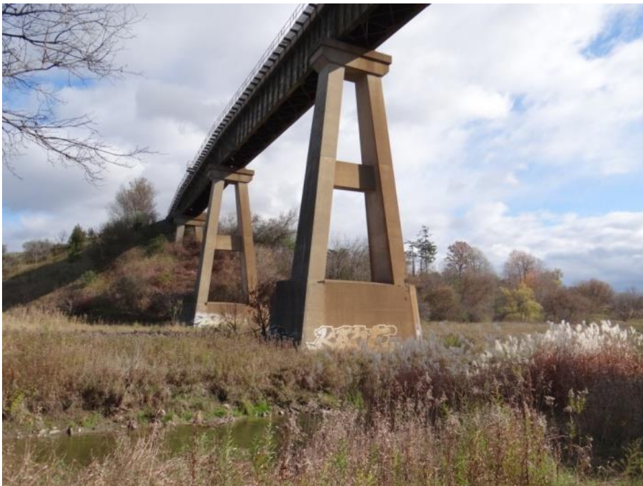
Plate 12: CN York Sub Bridge over the Humber River, south of the study area, looking south.
