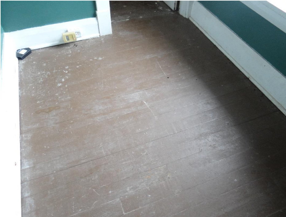
Plate 23: Detail of second storey wood floors
