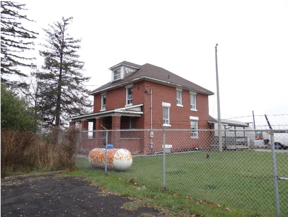
Plate 1: Front facade (east elevation) of the farmhouse
